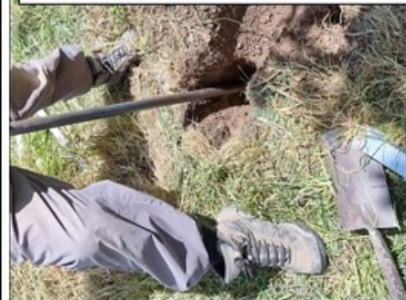
Digging the holes for H frame and posts
