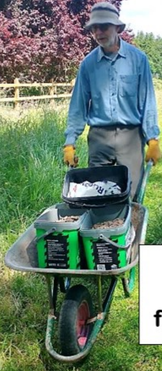
Arriving with the cement and ballast
