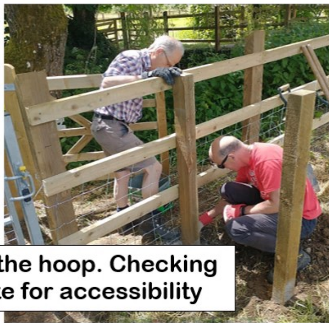
Metal gate now bedded in with hoop and fence formwork being constructed
